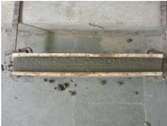
Fig. 4 Formwork prepared on site.
