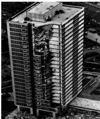
Figure 1. Ronan Point Collapse
