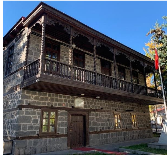
Figure 13. Wooden Balcony in Eastern Anatolian Architecture [10].
